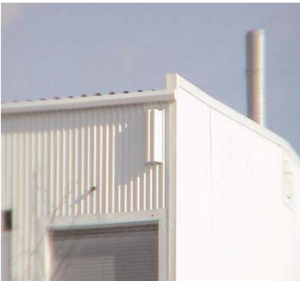
Figure 8 : A good example of an Antenna that has been camouflaged so as to minimise the environmental impact. (Source: 3G Website)
